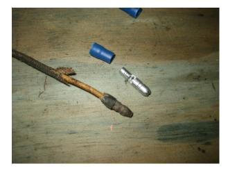
These were then crimped onto the new wiring.
